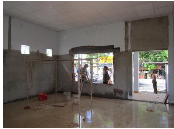
Conversion of old toilet block to beauty training centre
