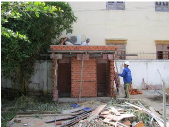
Construction underway on new toilet block at Long Hai
